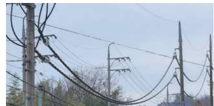
22.9kV Insulation cable installation site
